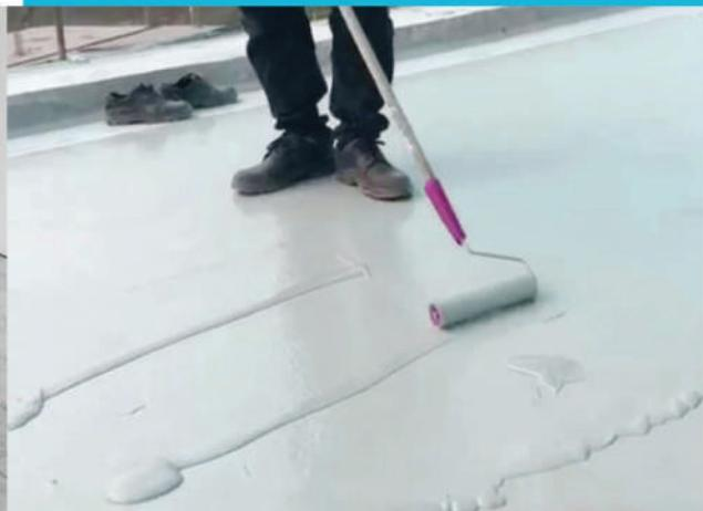
DAMP COAT EX 2000 is an advanced formula developed based on Acrylic Cementitious protective coating for water proofing of RCC roofing and bathrooms. It forms seamless, durable membranes with excellent water proofing protection. It is an environment friendly non toxic water proof coating providing strong adhesion and excellent durability.
